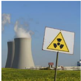
Energy: Nuclear Power Plants
